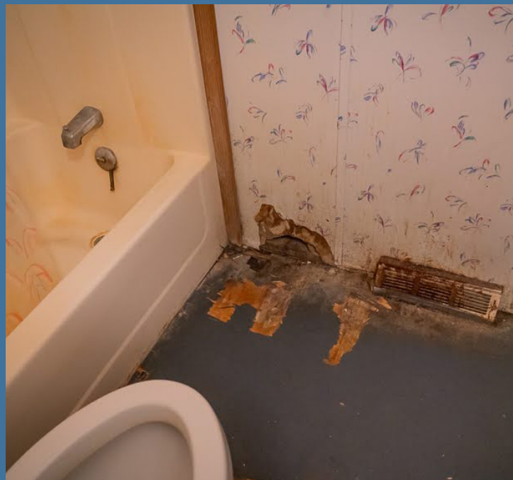
Before: Holes in the bathroom walls led to rodents entering the house. Exposed electrical wiring was a danger to the trailer's inhabitants. "No amount of scrubbing made it clean."
