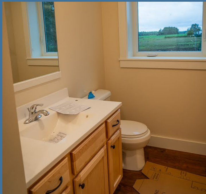
After: The new house has two bathrooms in pristine condition. The building's green design ensures a consistent supply of clean and hot water for workers' use.
