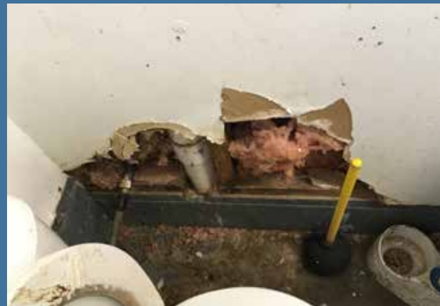
Before: Holes in the bathroom walls led to rodent infestations
